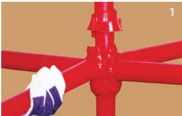
Fix ledger blade ends into lower cup
