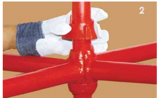
Position the upper cup over the top end of ledger blades
